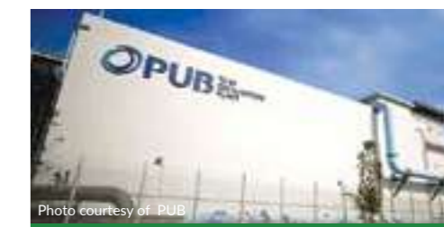
Tuas Desalination Plant Desalination Plant of the Year, Global Water Awards (2019)
