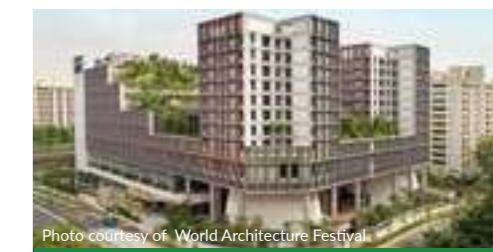
Kampung Admiralty Housing Project World Building of the Year at World Architecture Festival (2018)
